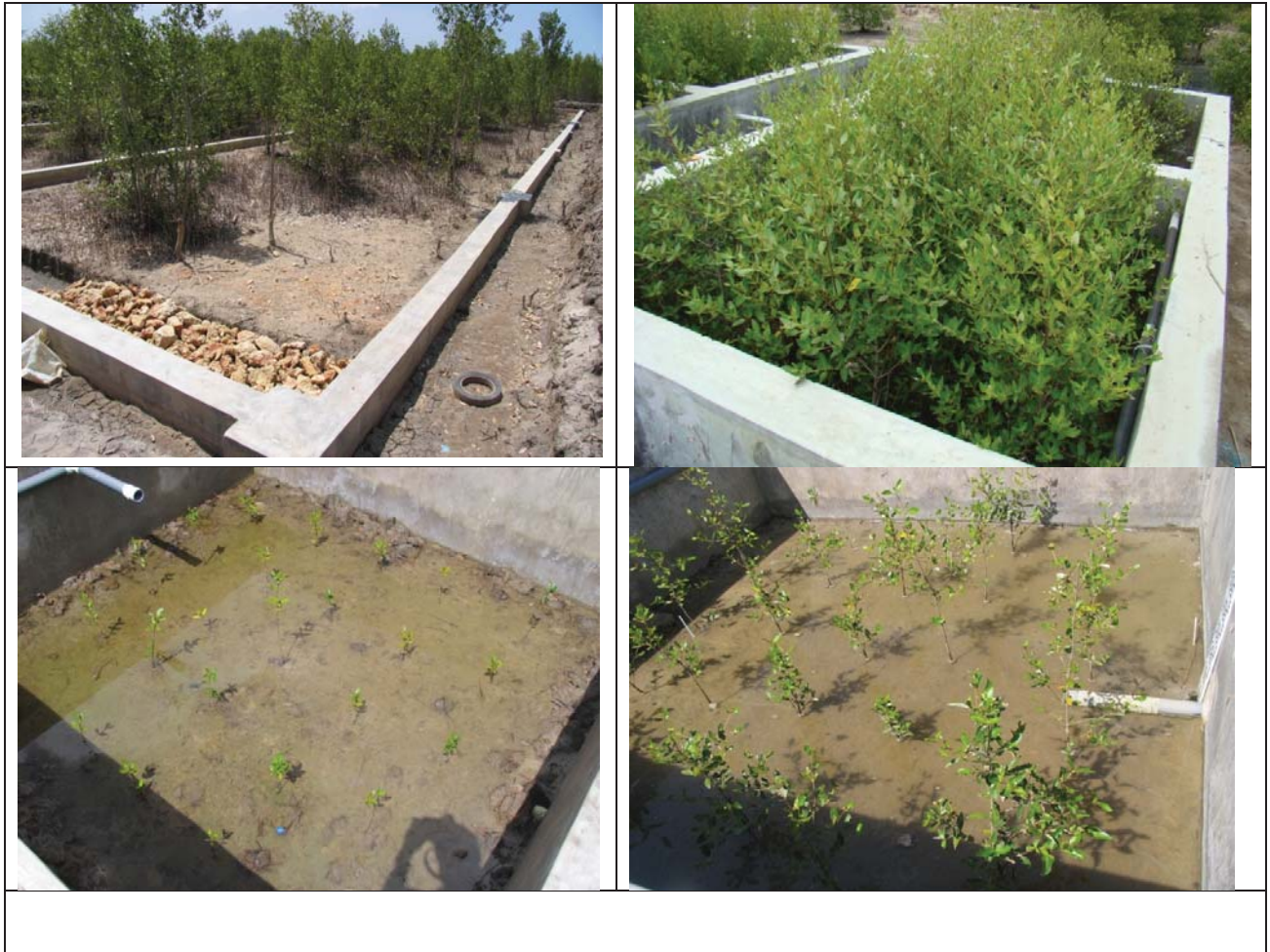
Figure 3: Mangrove Constructed Wetland
